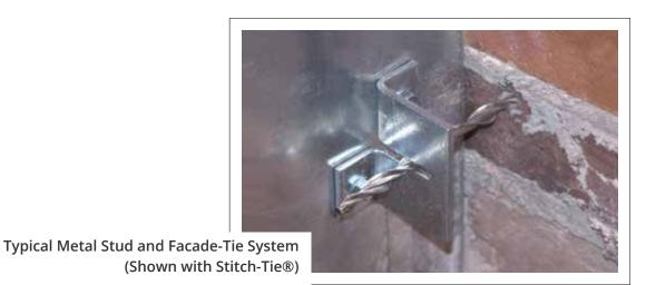
Whether the Stitch-Tie System or the Grip-Tie System is used, it WILL NOT pull the veneer material to the base structure. The primary goal is to stabilize the veneer from moving any further.
