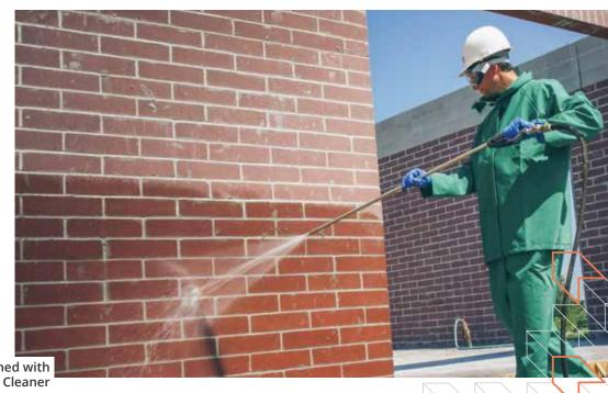
Concrete brick being cleaned with Light Duty Concrete Cleaner
